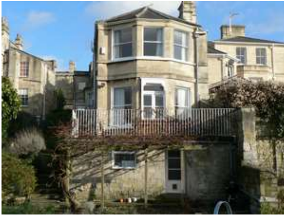
Canal view of No 9 as it is today
